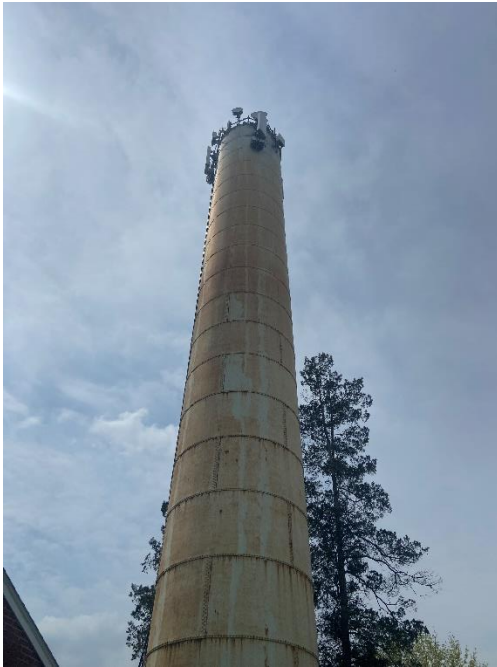
Standpipe with antenna and tree that will need removal.
